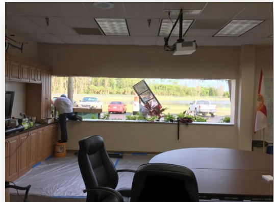
Removal of the old windows in the boardroom
