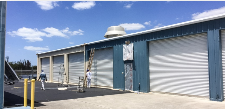
Vehicle storage building being painted
